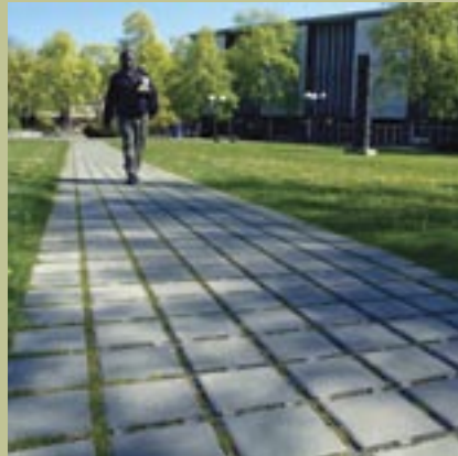
Permeable paving stones reduce stormwater runoff.
