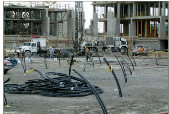
Figure 3: Installation of GHX Borehole Field
