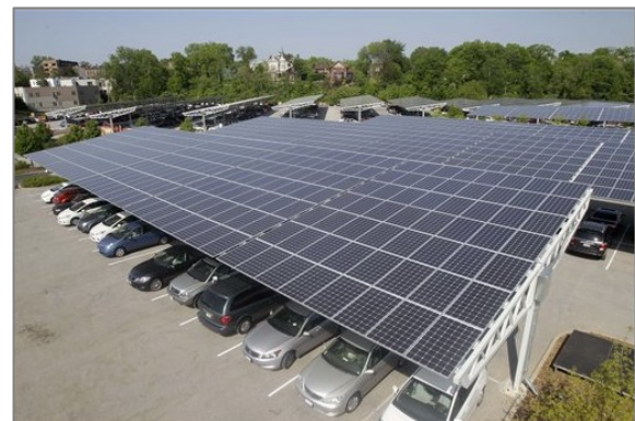
Figure 1: Example of a photovoltaic system integrated into car park shading
