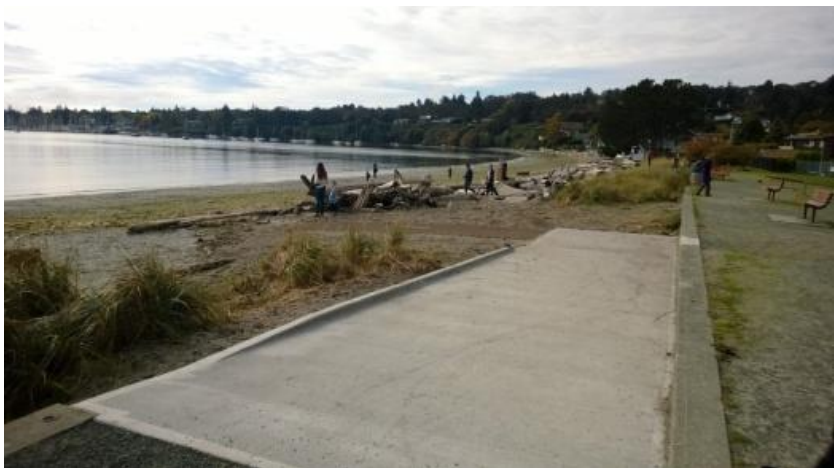
Figure 8: Newly commissioned mobility improvements include a concrete wheelchair ramp, as viewed looking southwest (Cox, 2013)
