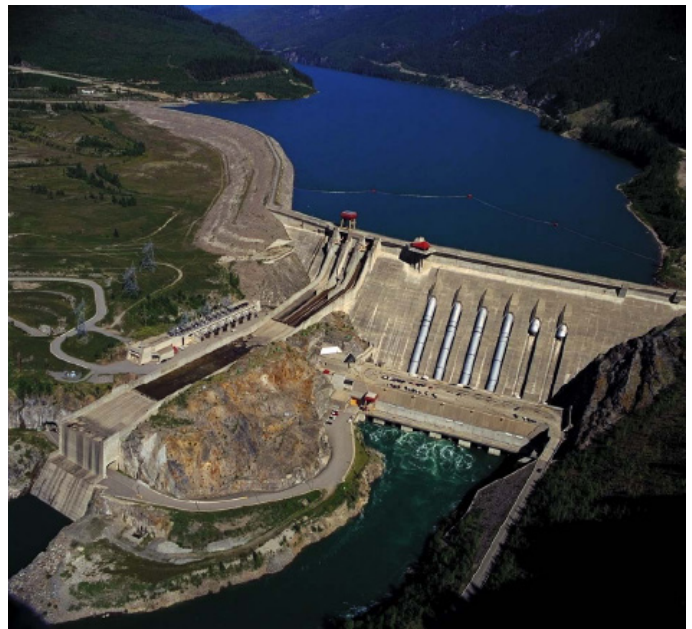
Figure 8-1 – Revelstoke Dam looking north
