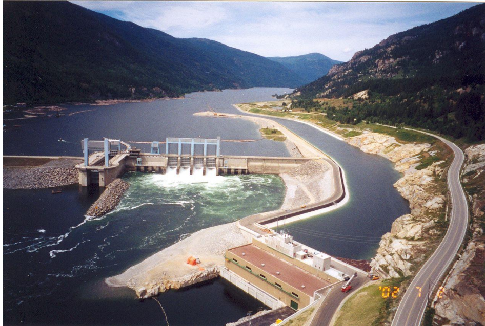
Arrow Lakes Dam, BC 185 MW capacity An average size of 68 dams in BC.
