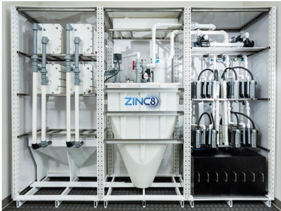
Figure 2.2 ZAFB system (image credit: Zinc8) [9]
