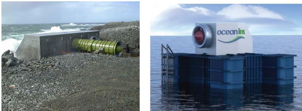
Figure 10: Devices based on the OWC principle. Land Installed Marine Power Energy Transformer (LIMPET) installed in Scotland by WaveGen 12 (left) and greenWave, a device designed by Oceanlinx 13 installed in Port MacDonnell, Australia
