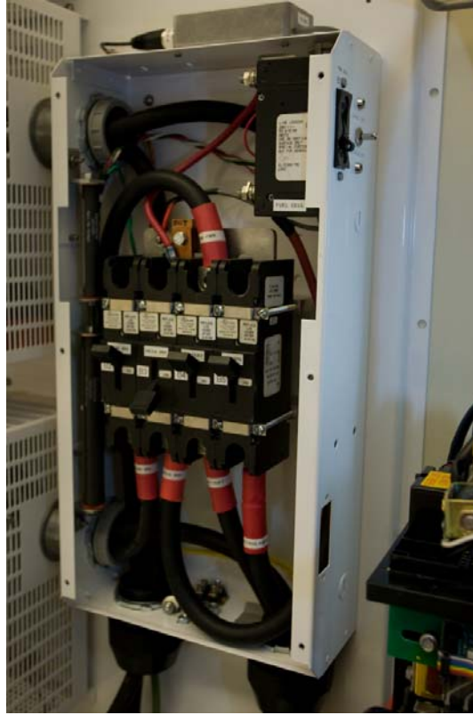
Figure 4.3 DC Bus Bar and Disconnects
