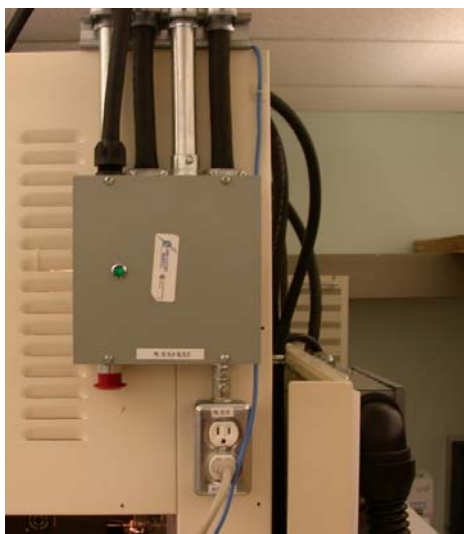
Figure 4.7 Emergency Shut Down Interface
