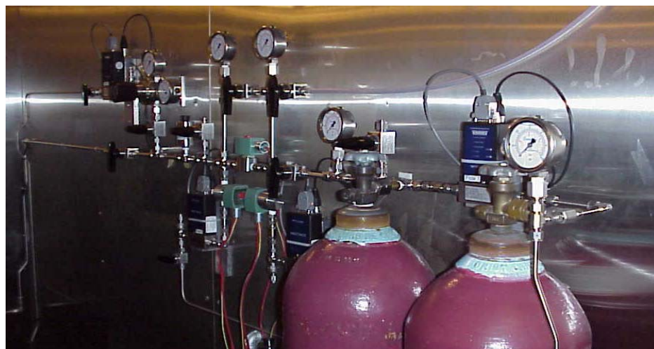
Figure 4.16 Fume Hood Hydrogen Distribution System
