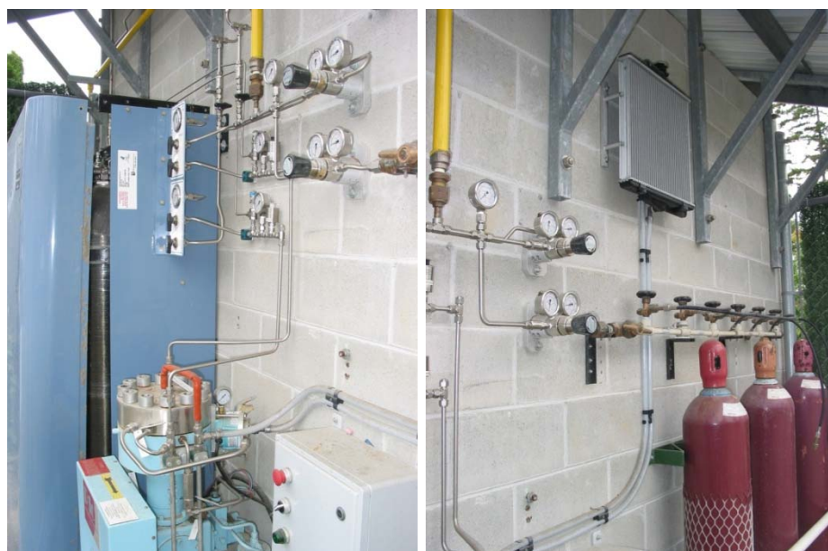
Hydrogen Compressor Installation
