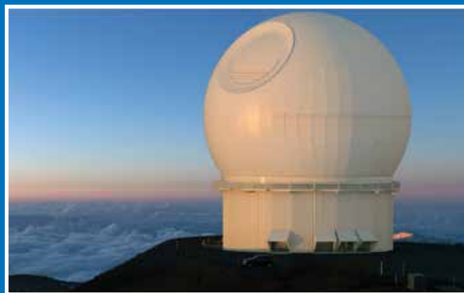
A rendering of MSE in the current location of the CFHT on Maunakea. The MSE dome is only 10% taller than the current CFHT dome, despite the telescope being nearly three times larger in diameter.
