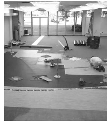
Renovations in progress at McPherson Library
