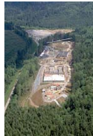
Seattle Public Utilities' Tolt Treatment Facility
