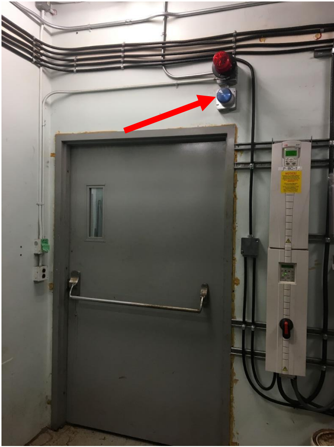
High and Low alarm lights in compressor room
