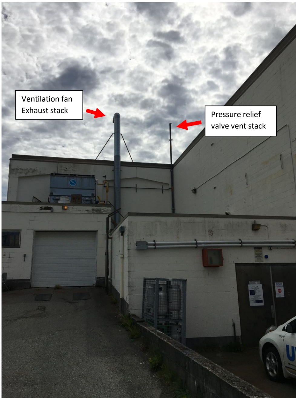
Emergency Pressure Relief Valves and Compressor Room exhaust stacks
