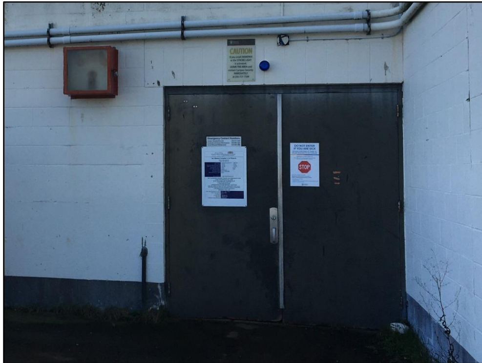
Figure 1: Entrance to Electrical Room. Blue alarm light and warning located above door
