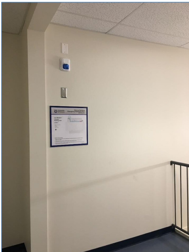
Figure 8: Alarm indicator light upper floor stairwell
