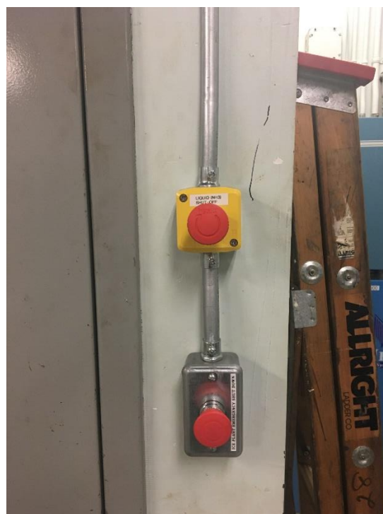
Emergency shut down switches for Ice Plant
