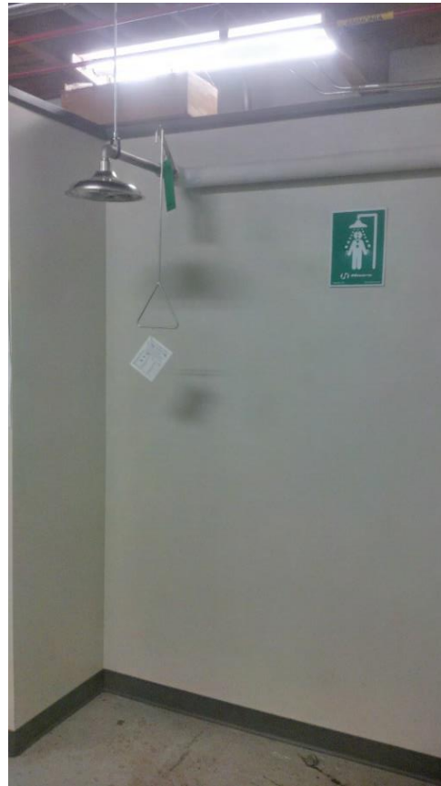
Emergency Shower in front of Compressor Room
