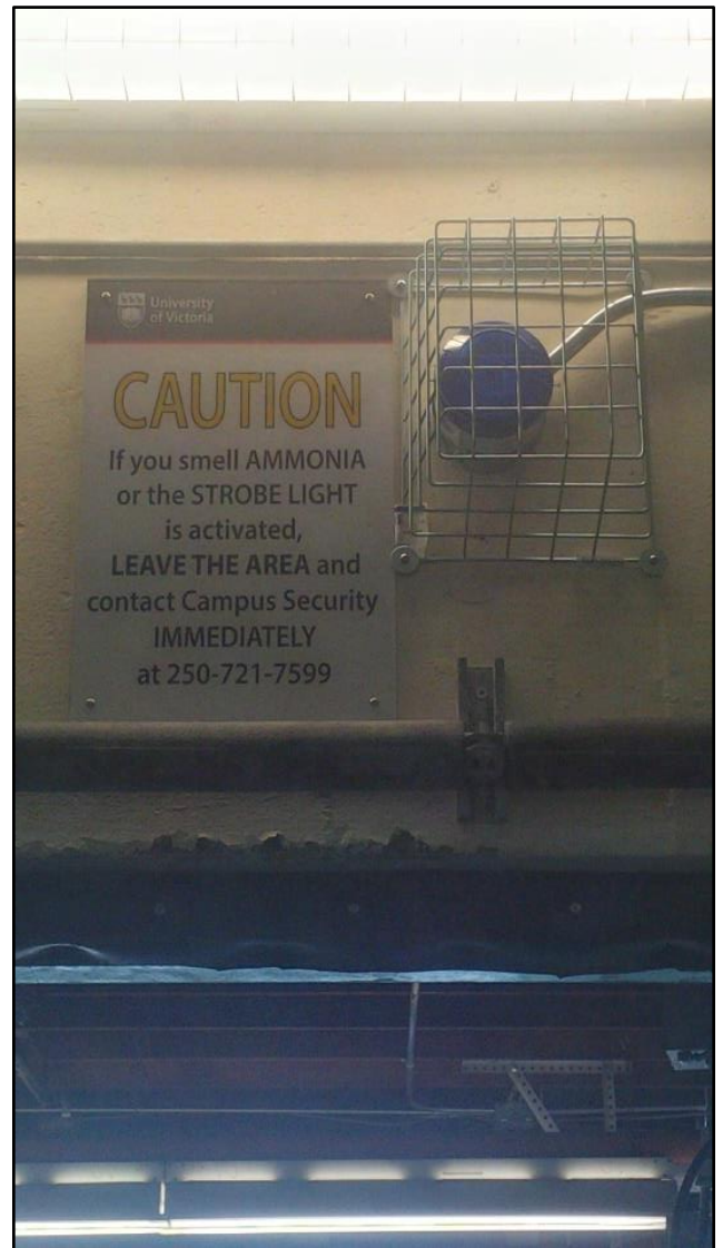
Figure 5: Alarm indicator light and warning sign over interior Zamboni room door
