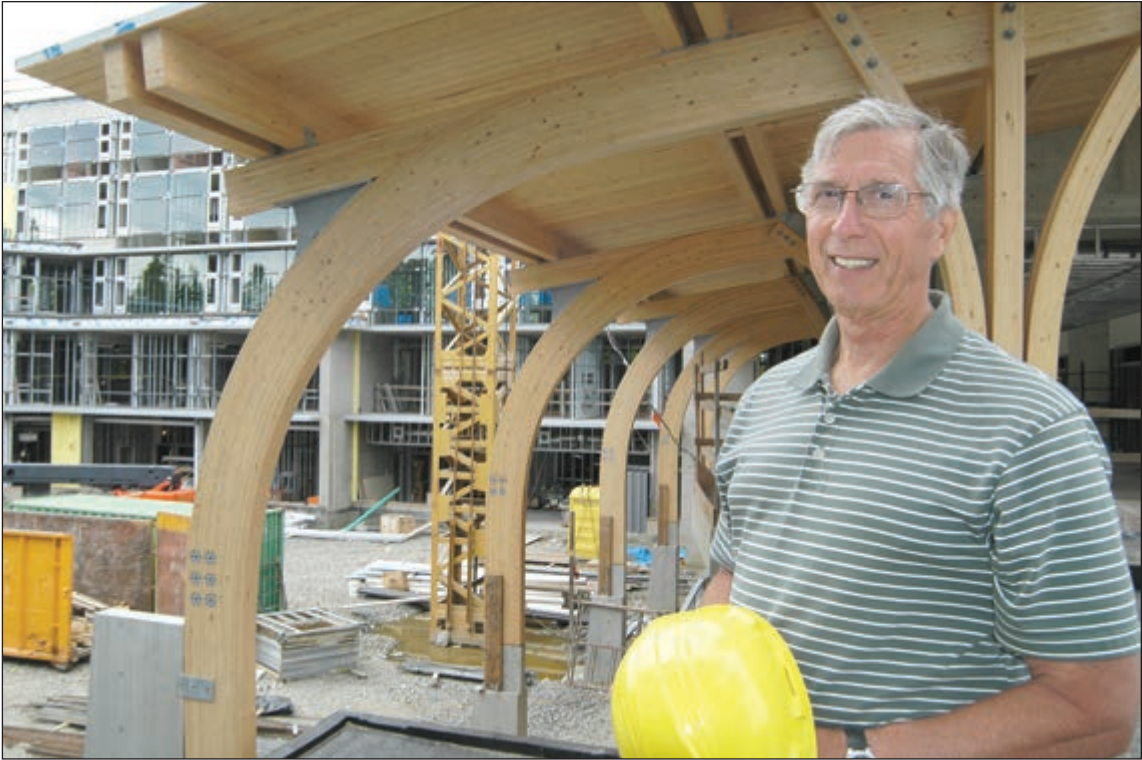
Facilities Management Project Officer Bruce James shows off the arching columns at the front entrance of the new Social Sciences and Mathematics Building. Made from laminated beetle-killed pine, the columns are one of many sustainable features in the new building.
