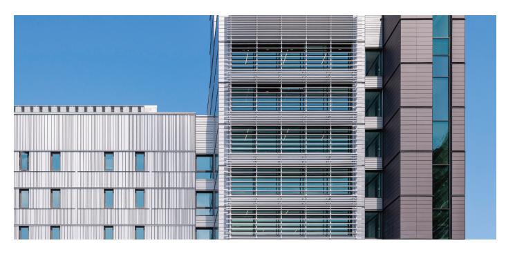
To optimize access to daylight and energy efficiency, window ratios are balanced to meet thermal performance targets, allowing for generous floor-to-ceiling windows in public areas.
