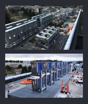
The new buildings capture this waste heat using Heat Recovery Ventilation (HRV) devices, and re-use it to warm incoming fresh air, significantly reducing the energy used for space heating in each building.
