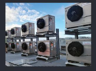
Electric Air Source Heat Pumps are being used to heat water in both buildings instead of natural gas energy from the District Energy System. In addition, the pipes transporting water will be shorter in length and have increased insulation to minimize heat loss. The combination of these strategies will result in an 88% reduction of GHGs associated with the process of heating water.
