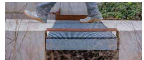
Example of perforated surfacing for water filtration into wetland
