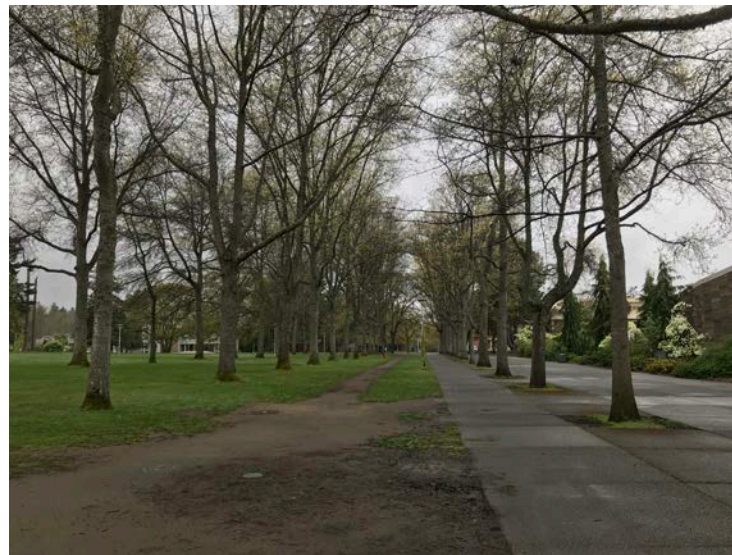
Evidence of new pedestrian routes being established as a result of insufficient pedestrian flow management and pathway width.
