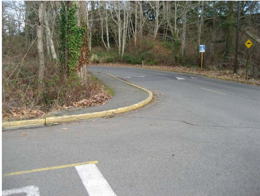
FIGURE C-7 WEST CAMPUS WAY AT LOT 9 ACCESS FACING NORTH The horizontal curve and surrounding shrubbery results in poor sightlines for vehicles exiting Lot 9.
