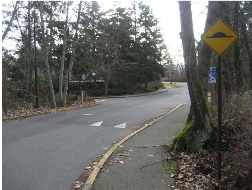
FIGURE C-8 WEST CAMPUS WAY AT LOT 9 ACCESS FACING SOUTH Speed humps are generally effective in slowing vehicles. However, the southbound speed hump and accompanying sign are after the horizontal curve and might not be seen until late.
