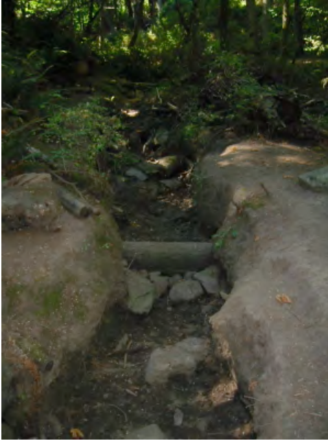
Figure A-1. A weir installed by UVic to trap sediment in a downcut section of Hobbs Creek.
